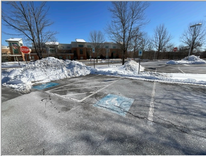
OVERVIEW OF ACCESSIBLE PARKING AREA
